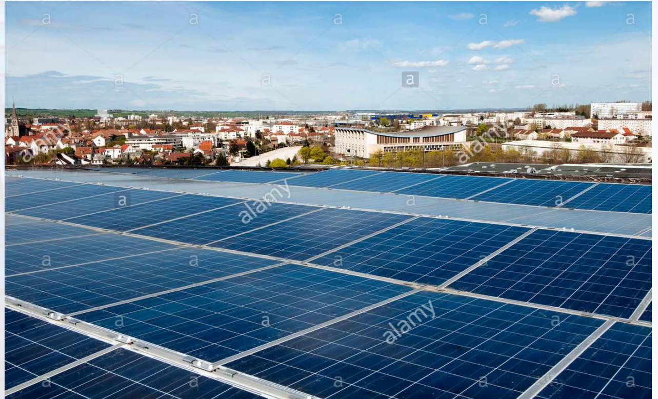
Horizontally tilted solar panels
